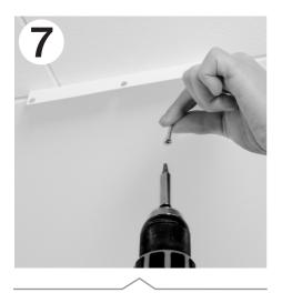
Mount the roof bracket with the supplied wooden screws. (Other attachment may be required for porous material).
