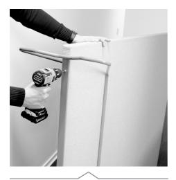
Fit the sound absorber in place on the frame using the 3 wood screws supplied.
