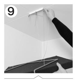
Use the wire locks in the hooks to adjust the length and angle.
